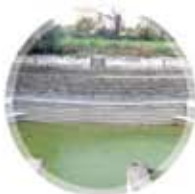
Rain Water Harvesting and Drip & Sprinkler Irrigation
